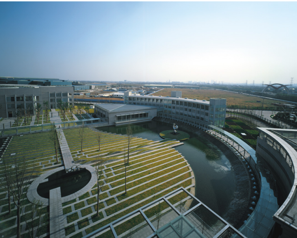
Industrial & Commercial Bank of China—Data Center Wai Gao Qiao Free Trade Development Zone, Shanghai, China Joseph Wong Design Associates (JWDA Ltd.)
